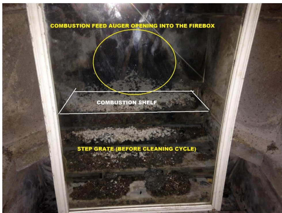
Figure 32 Evoworld HC 100 combustion chamber with grass pellet residue, March 2015
