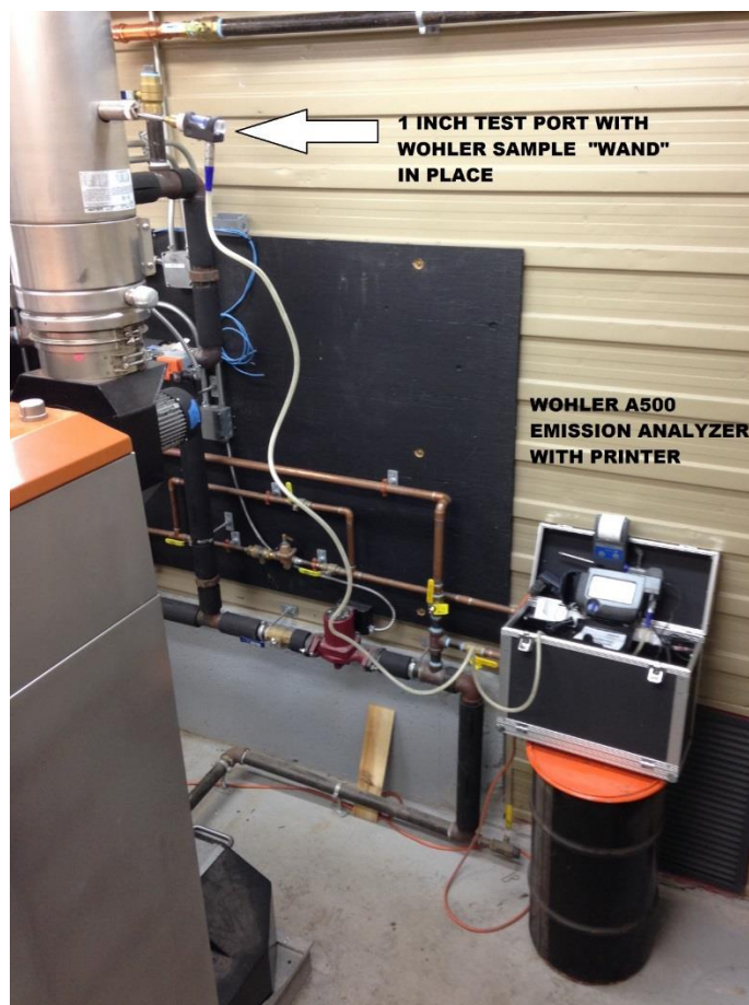
Figure 28 Wohler A500 set-up to sample, March 2015
