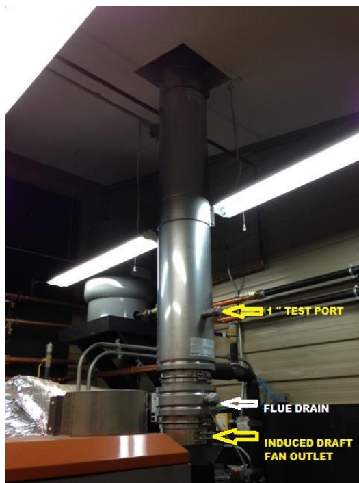
Figure 9 Evoworld HC 100 Eco boiler - 8" flue showing test port, 6-23-2015
